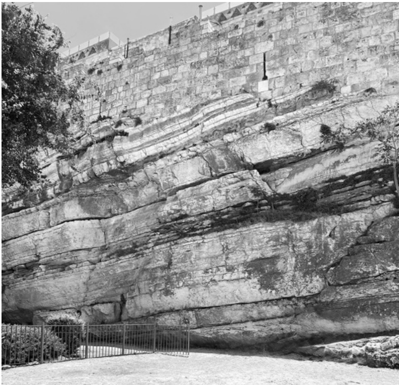
Section of the wall set on top of a quarried cliff east of the Damascus Gate of the Old City, Jerusalem
