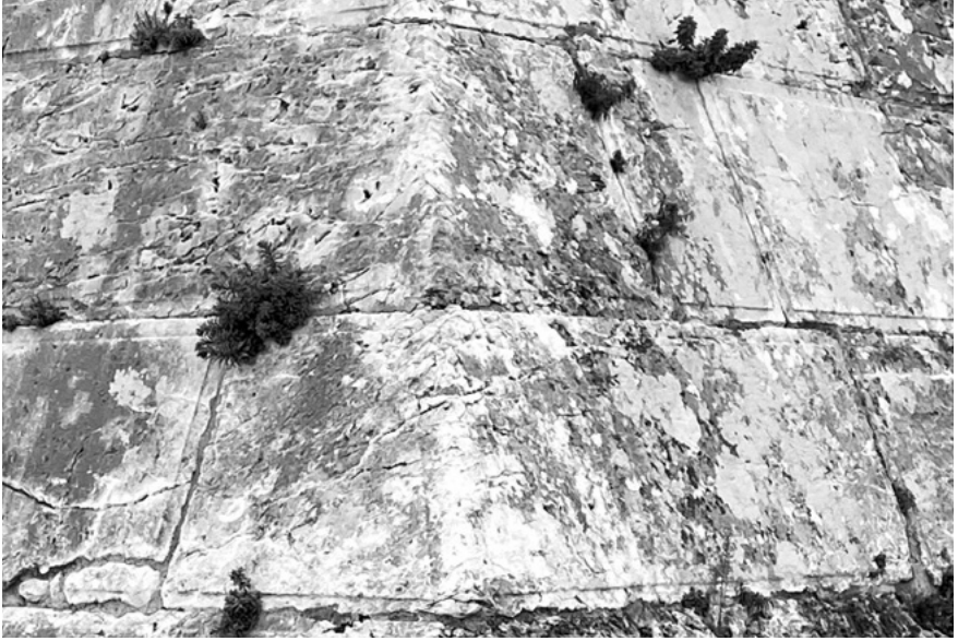
Close-up of the defensive corner of the Tower of David built with large, fine ashlars with chiseled margins.
