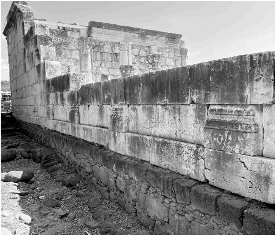
Capernaum synagogue on a basalt foundation with fine limestone ashlar above with carved pilasters like those seen in Jerusalem.
