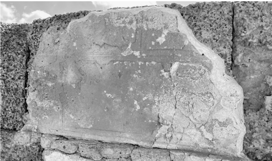
The plaster over the stonework at Caesarea was again carved to look like the ashlar stones of the Temple Mount.
