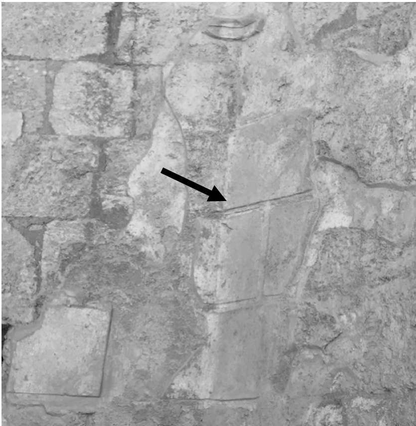
A plaster remnant over Herod's stonework at the Herodium that was carved to look like bordered ashlars is seen here (arrow).
