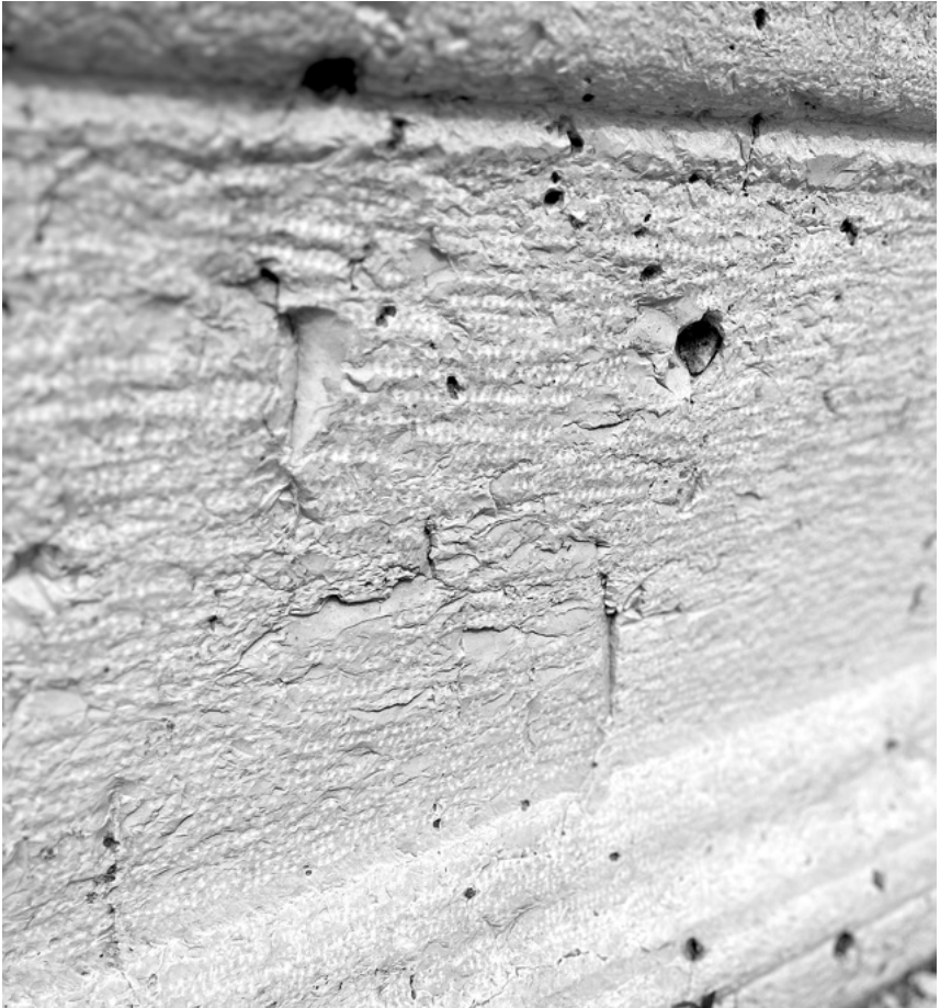
Chisel marks on fine limestone ashlars at Sebastia
