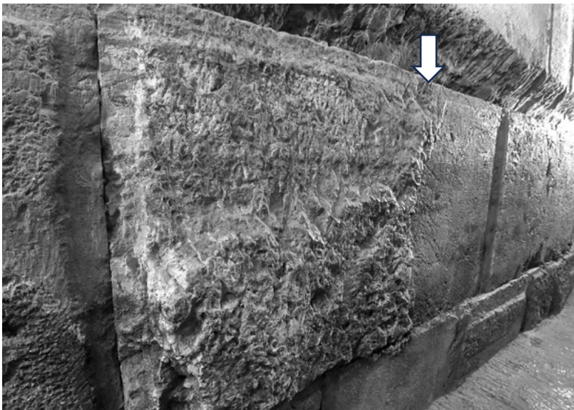
A single ashlar stone where only half has been finished with a smooth front (a white arrow marks the transition).
