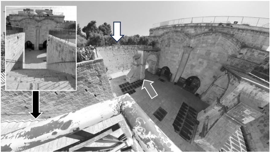
Excavated Golden Gate with retaining walls to protect it (white arrow), entrance stairs (black arrow), and arches (gray arrow) that were added to support the walls of the gate in 1892.
