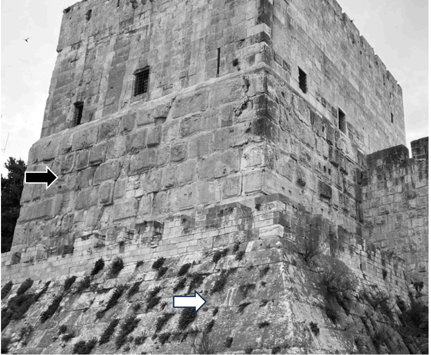
Tower of David with smooth faces like the Temple Mount (white arrow) and large ashlars with rough faces (black arrow).
