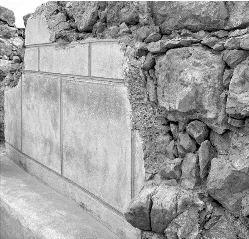
Plaster veneer over stone carved to look like fine drafted ashlar stones at Masada.
