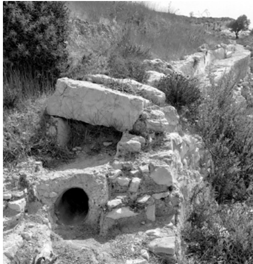
Section of the aqueduct between Solomon's Pools and Jerusalem
