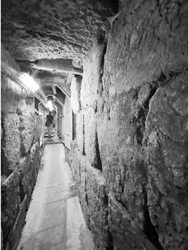
Drain channel section that runs over 650 yards from the temple area down past the Pool of Siloam.
